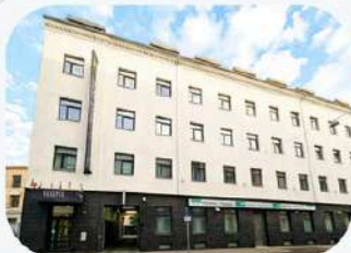
EFI Palace, Brno
